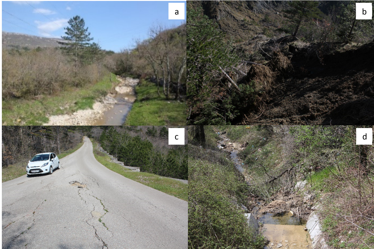
Figure 3: (a) Sediment in tributary Malenica riverbed, (b) Land instability: intensive erosion processes causing local landslides on Slani Potok sub-catchment (c) Road damage due to land instability on border of Slani Potok and Mala Dubračina sub-catchments, (d) Unmaintained river bed of one of the Dubračina tributary's [photographs taken by author]
