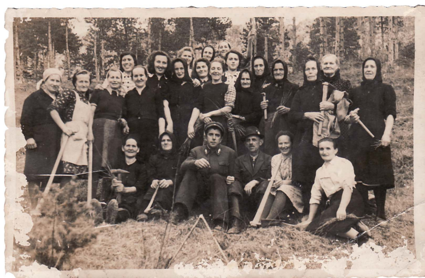
Figure 5: Local population involved in mitigation measures: reforestation of erosion affected areas (source local inhabitants archive)
