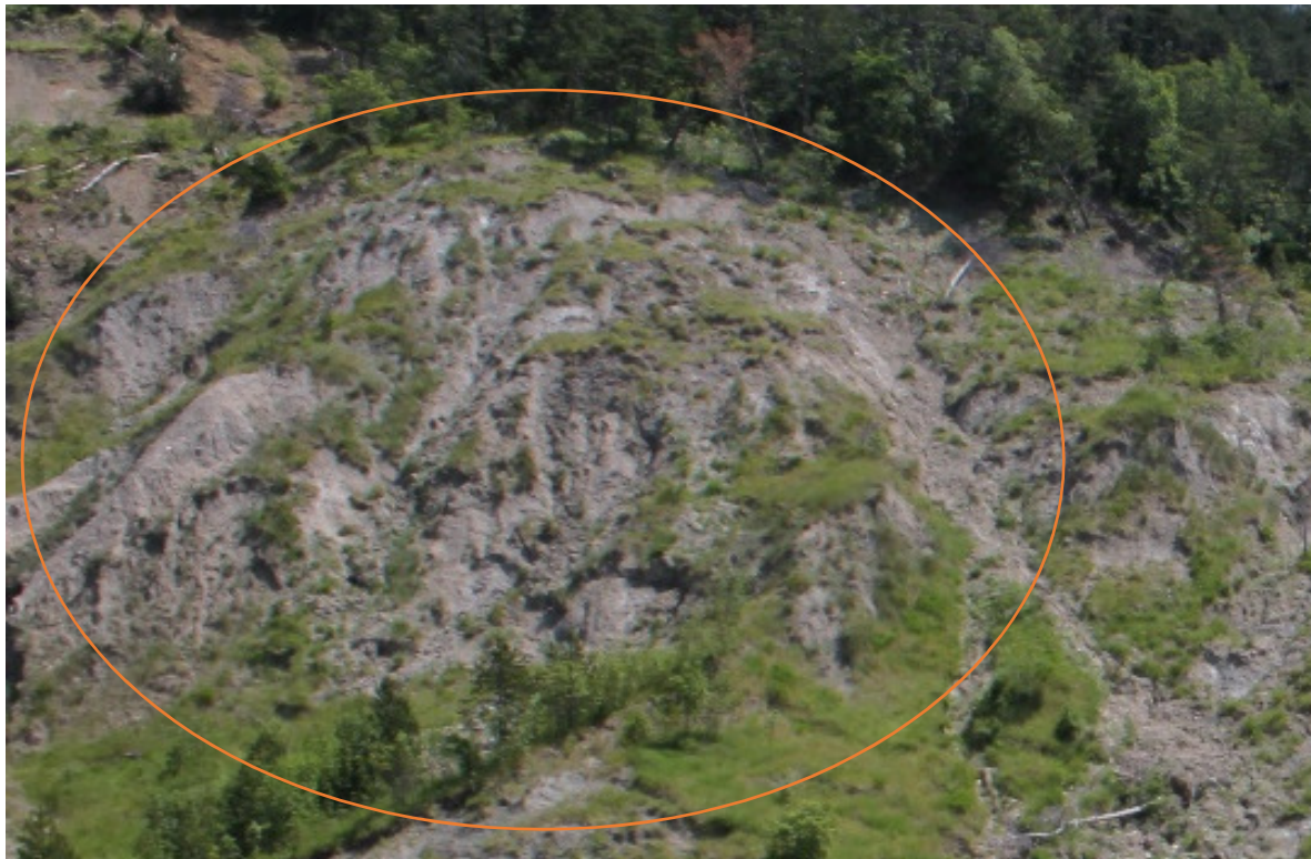
Figure 51: Location used for close range photogrammetry measurement method (photograph taken by author in June, 2014)
