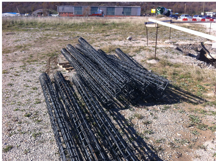
FIGURE 5.3: Pile reinforcement cross-section
