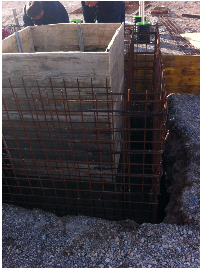
FIGURE 5.10: Counterweight block reinforcement
