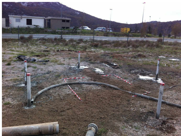
FIGURE 5.7: Inclinometer casings arranged in test field
