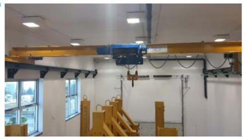
Short description Single girder bridge overhead crane SPB INŽENJERING d.o.o. type JMD 5t/8,583m with crane runway length 16 m
